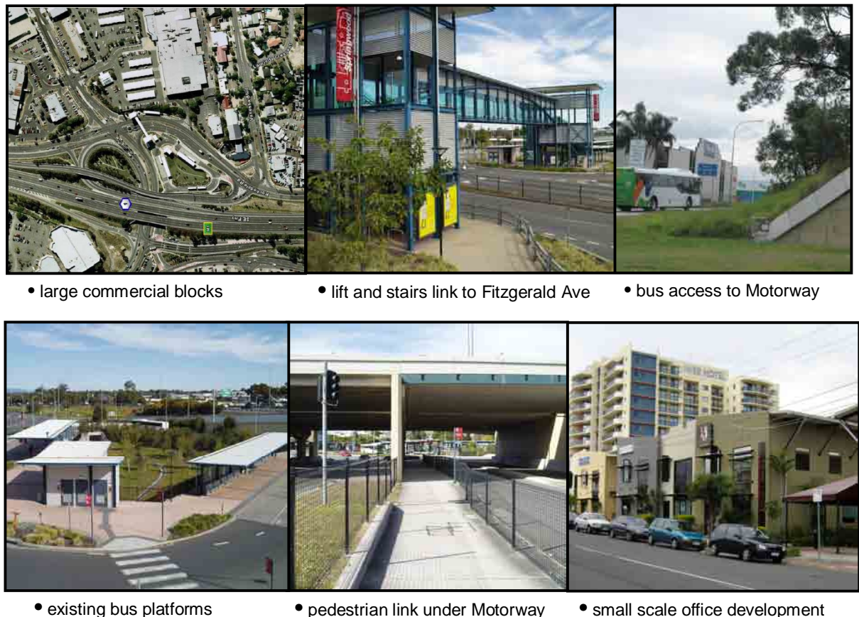
Figure 6-3: Existing urban environment — Springwood
